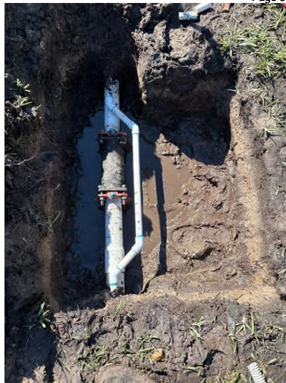
Mainline repair along Ayersworth
