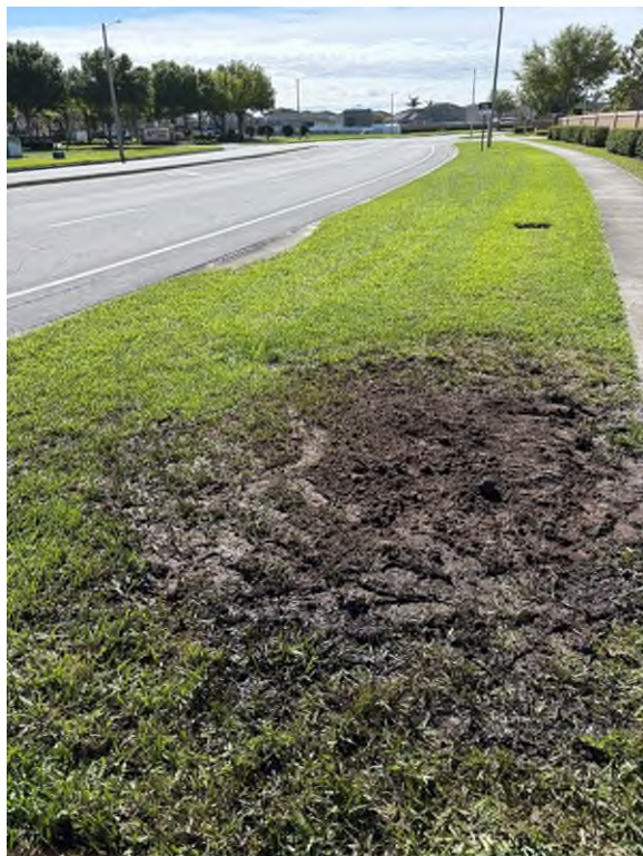
Mainline leak along Ayersworth
